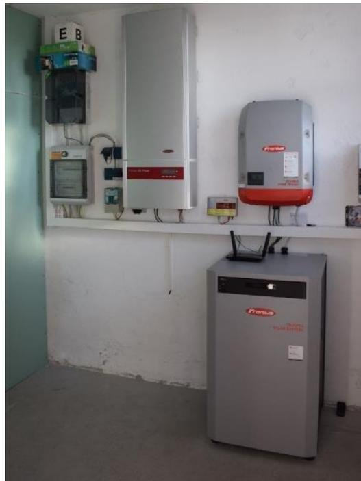
**Figure 16: Implemented PV system together with the PV-BESS at the customer premise**
