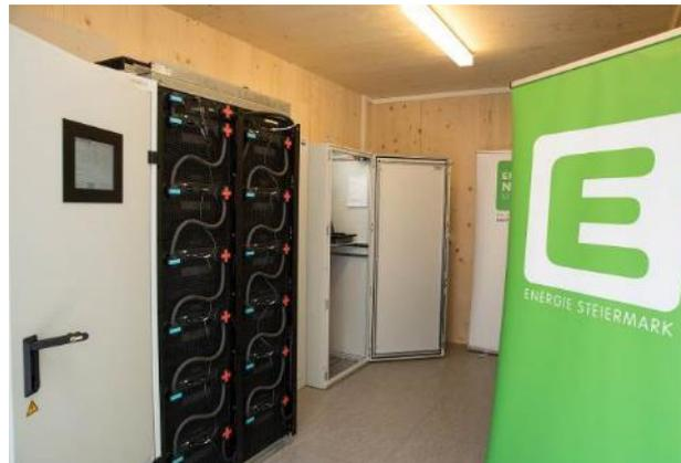
**Figure 24: Inside view of the Urban Box: Inverter (left), Battery (centre), controller (right)**
